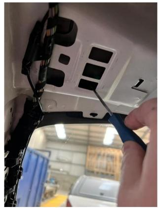
Fix lightbar bracket to the <u>top</u> of mounting bracket with fixings fitting from the underside as shown below. (Use assembly drawings for fittings reference)
