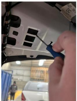
Place the mounting bracket on van roof like shown and place a bolt through the bracket hole and newly drilled hole in van roof.
